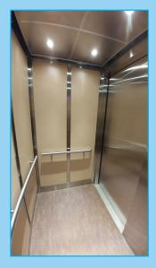
An elevator cab upgrade is optional when an elevator is modernized. The upgrade reuses the existing car and platform and sets new wall panels on the supporting shell structure that are separated with stainless steel reveals. As well, the face of the car and the front transom are capped in stainless steel and the hand railings are replaced to suit the current Code.
